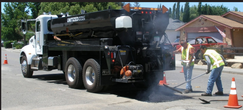
Compact asphalt material.
